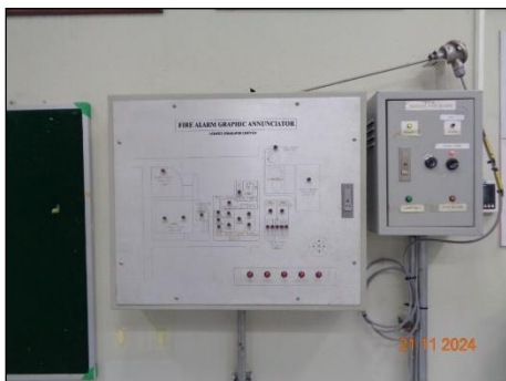
Fire Alarm Graphic Annunciator
